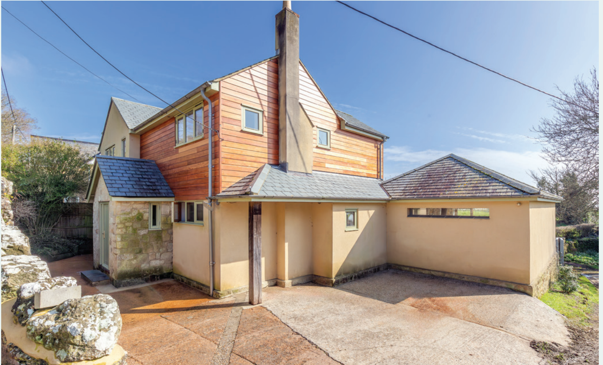
Ashmead, Sandrock Road, Niton, Isle of Wight
